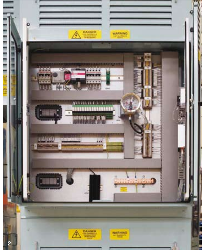
1. Diode bridge | 2. Terminal box of auxiliary connections | 3. Complete diode module (diode, heatsink and RC circuit) 4. Control box of the rectifier
